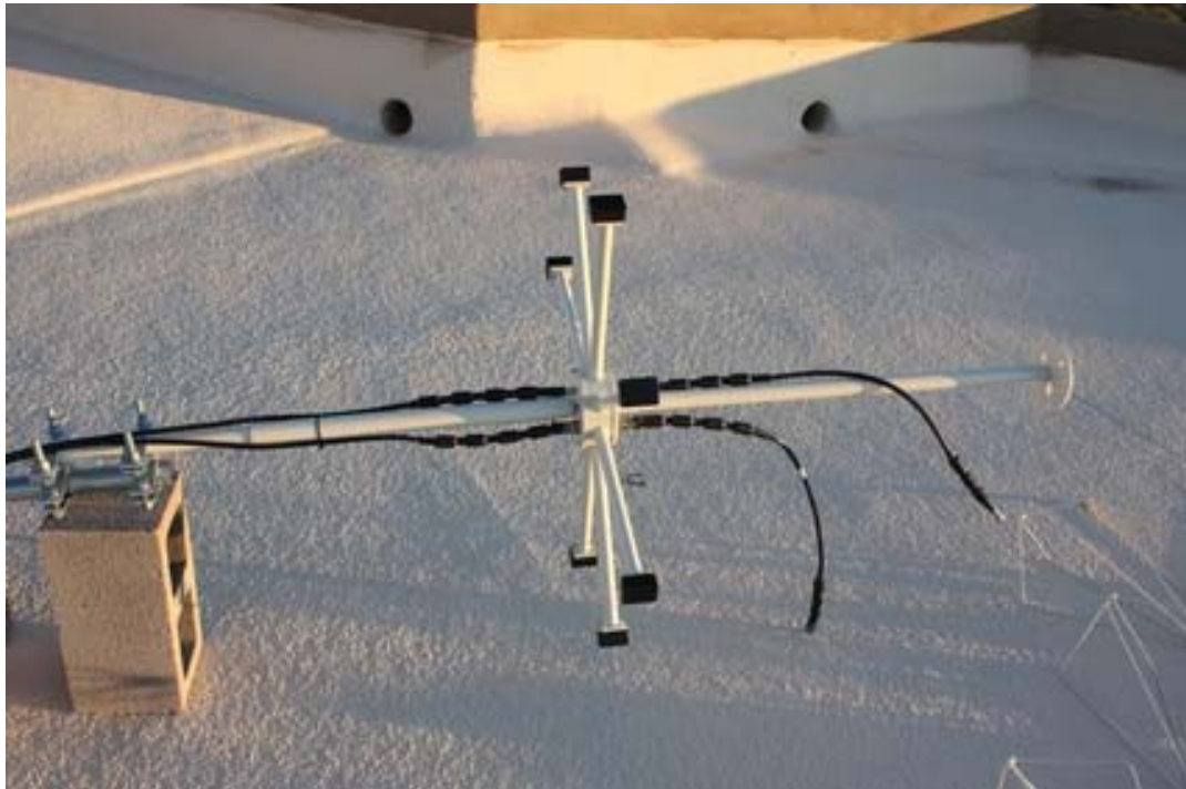
Figure 10: Connecting mast and cables installed for two antenna installation
